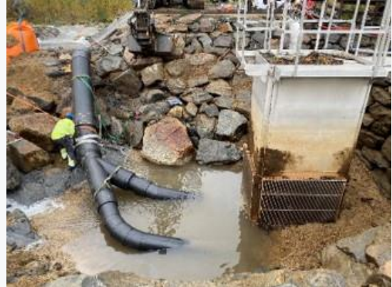
Sediments are removed from two sides
