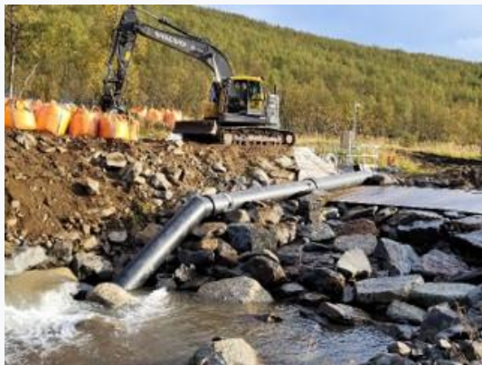
Installation and successful testing
