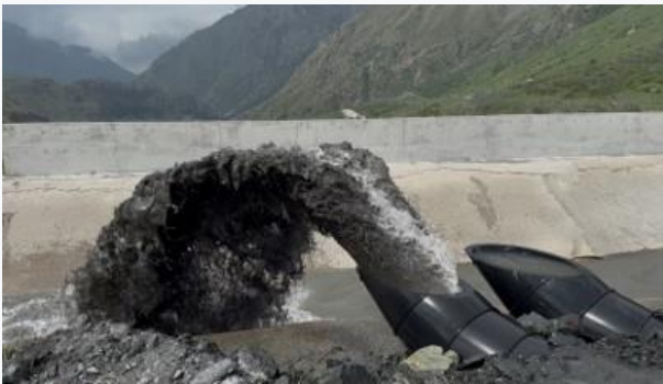
SediCon Sluicer discharging sediment from the forebay
