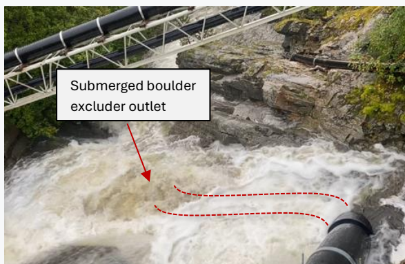
Sediment Excluder operating during flood conditions, September 2025
