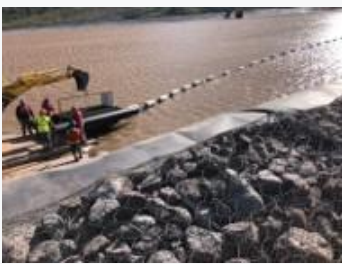
Floating pipe and barge arrangement at reservoir site
