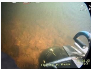
Dredging in fully submerged tunnel
