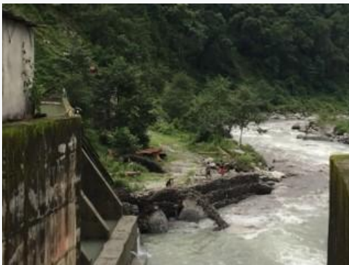
Outlet of SediCon sediment removal system
