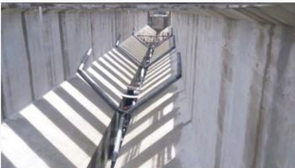
SediCon Sluicer installation
