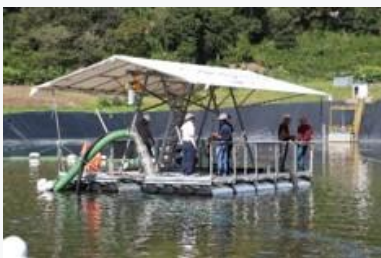
Remote operation platform
