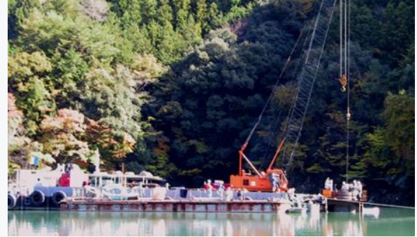
12x30m barge in Sakuma Reservoir
