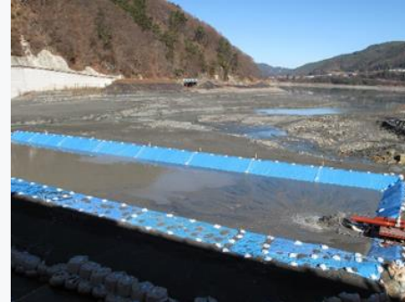
Full-scale SediCon Sluicer installed at Miwa Dam
