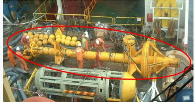
Pile Suction Head at Valhall Water Injection Project
