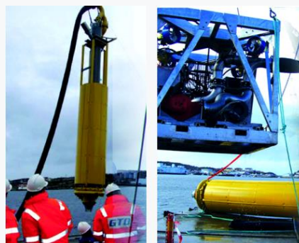
Pile Suction Head prepared for offshore deployment
