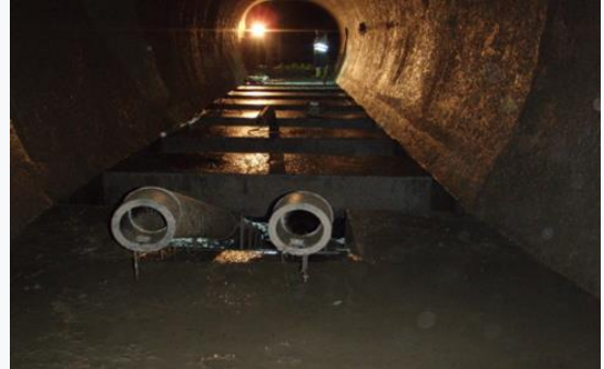
SediCon Sluicer installed inside the pressurized tunnel
