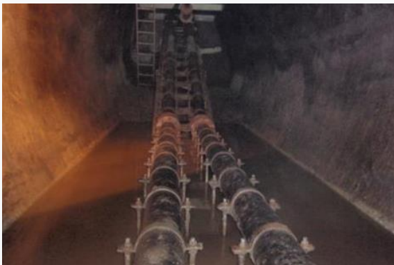
Sediment outlet pipes from the tunnel sand trap
