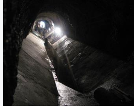
Pressurized desander during construction
