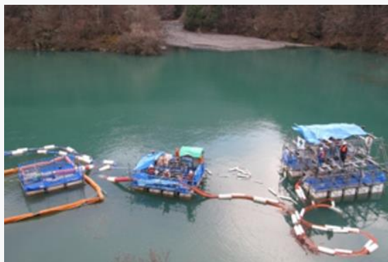
Floating work platform during dredging operation
