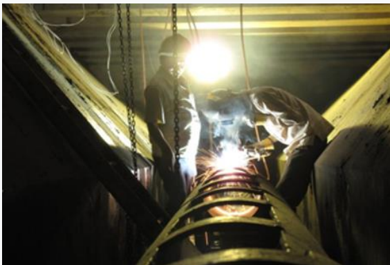
Installation of four SediCon Sluicers in the desander
