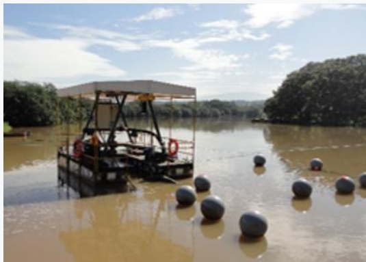
SediCon HydroSuction Dredge in operation
