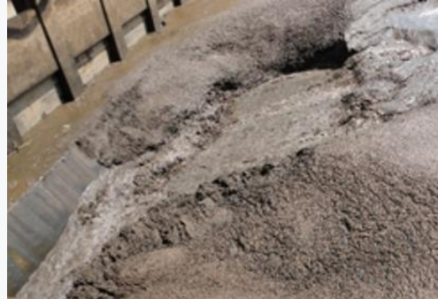
Sediment accumulation prior to dredging
