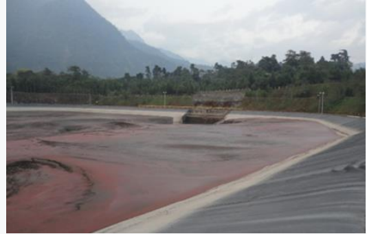
Forebay before continuous dredging (January 2012)
