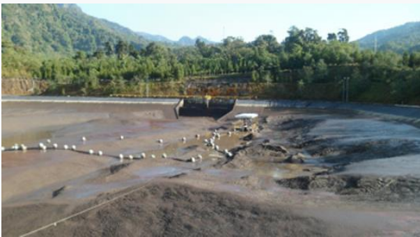
Forebay after sediment removal (February 2012)
