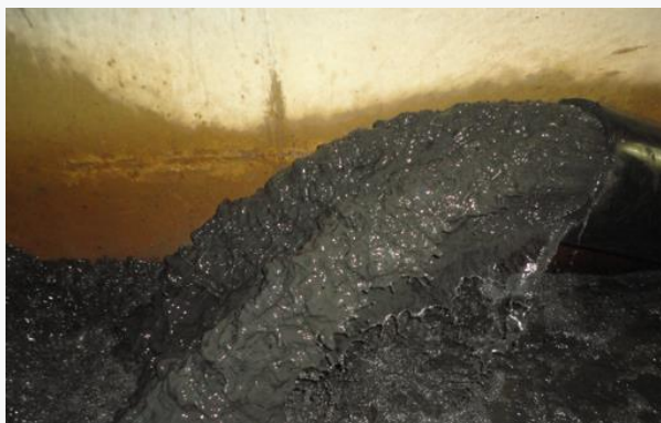
Sediment discharge during HydroSuction dredging
