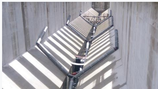
One of eight desanders equipped with five SediCon Sluicers each
