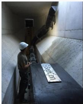
Ø355 SediCon Sluicer installed in the desander
