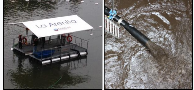
SediCon HydroSuction Dredge and Sediment discharge
