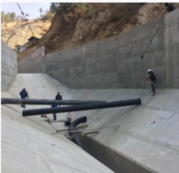
Installation of SediCon Sluicers
