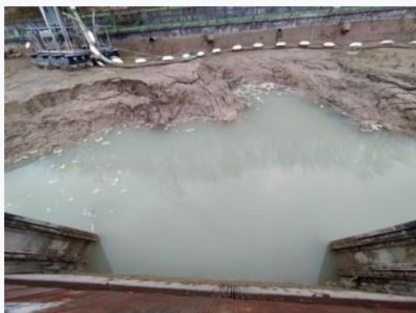
Dredging of Arlia reservoir
