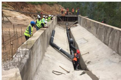
Installation of the SediCon Sluicer system
