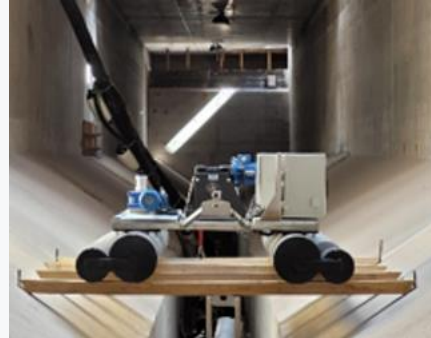
Installation of Desander Dredge in Alfalfal II desander
