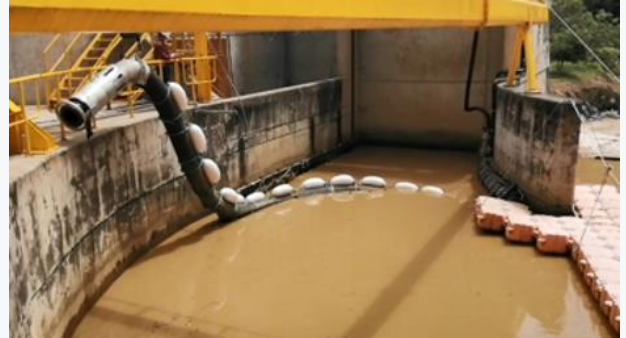
SediCon HydroSuction Dredge
