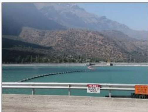
Pipeline in Las Lajas reservoir
