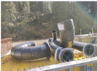
HDPE components & combined Sluicer outlet and spillway
