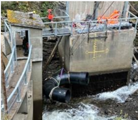
Challenging installation in a narrow gorge!
