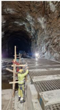
Downstream desander with 4 SediCon Sluicers
