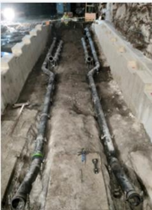
Downstream desander with 4 SediCon Sluicers
