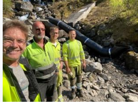
SediCon team and client during installation
