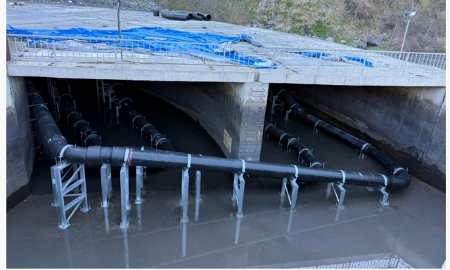
Dariali HPP intake and SediCon Sluicer installation
