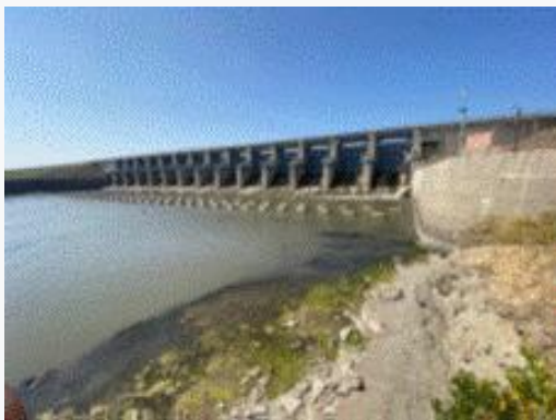
John Redmond Reservoir and dam outlet structure
