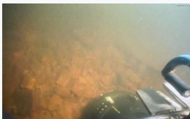
ROV-operated Ejector Dredge in a similar application
