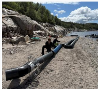
Preparing the SediCon Ejector Dredge and 250 m pipe system
