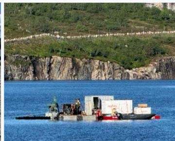
Surface raft with pump, pipework and ROV facilities
