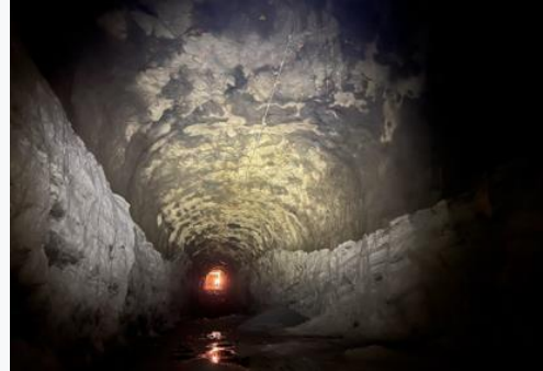
Svartisen Power Plant
