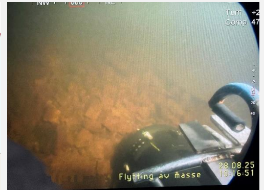
Dredging in pressurized tunnel
