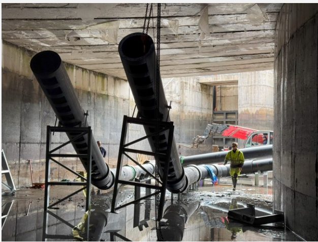
630 mm SediCon Sluicers remove sand gravel and stones up to 300 mm. Picture to the right is taken after two weeks of operation and shows that all sediment is removed.
