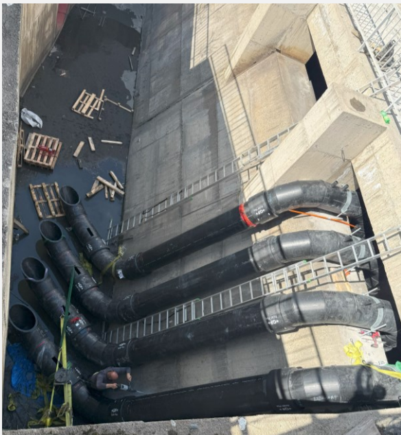
Four SediCon Sluicers discharge over the spillway. A starter system operated by a small water pump allows operation without valves and without any modification of existing structures.
