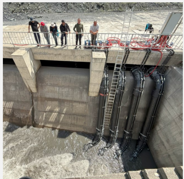
Four SediCon Sluicers discharge over the spillway. A starter system operated by a small water pump allows operation without valves and without any modification of existing structures.
