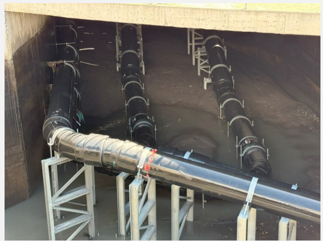
630 mm SediCon Sluicers remove sand gravel and stones up to 300 mm. Picture to the right is taken after two weeks of operation and shows that all sediment is removed.
