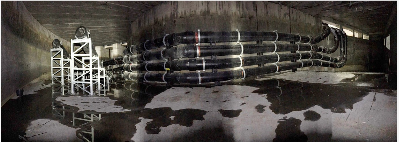
SediCon Sluicers in the intake. Outlet pipes along the wall discharge over the spillway.
