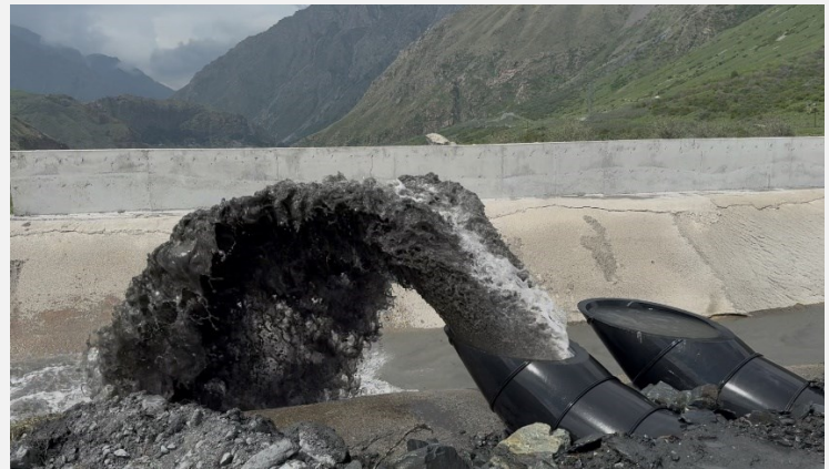
Discharge from SediCon Sluicers in the desander forebay
