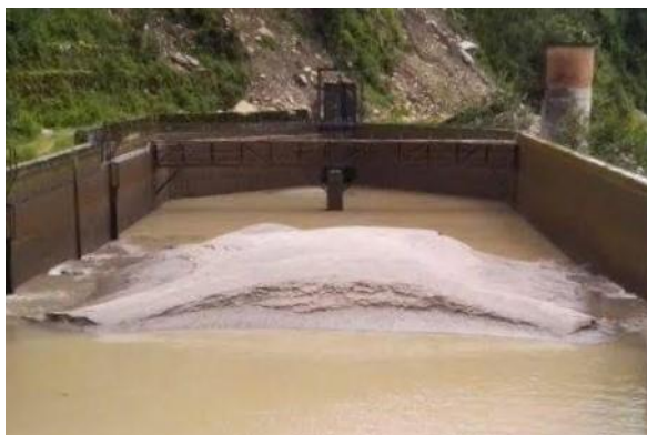
a) Sediment deposition prior to installation of SediCon Sluicer (Source: NHPC)
