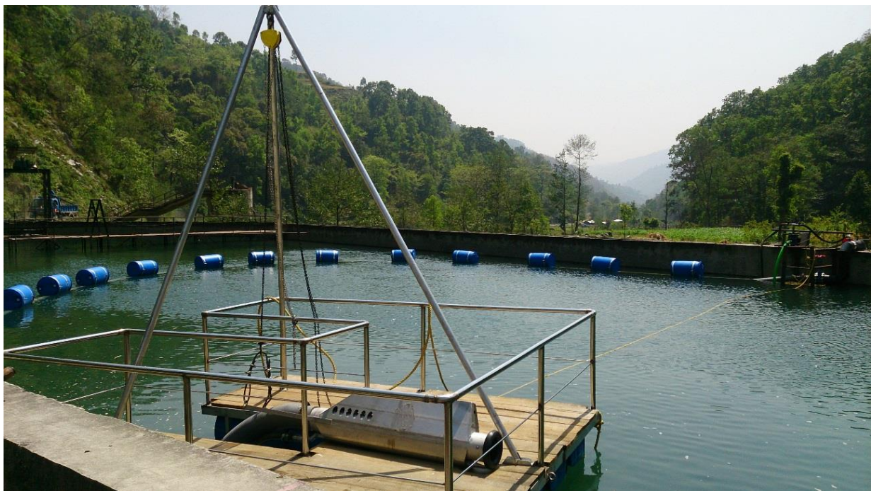
Fig. 5 SediCon Dredge at Indrawati III
